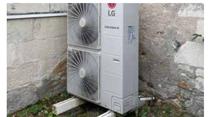
Example of a heat pump installation
